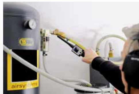
Leak detection with focus tube
